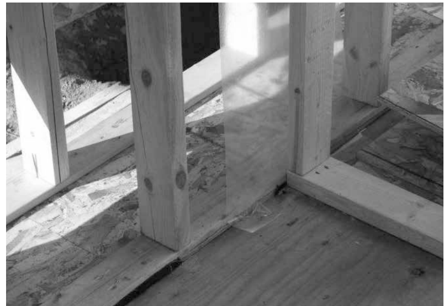
A double-stud wall system showing heat transfer improvement
